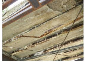
Both end sections of the deck have dropped together with the floor beams on the bearing seats as the floor beams are completely detached from the truss (failure of these deck sections could trigger collapse of the entire superstructure). The east section of the deck is in an advanced state of deterioration.
