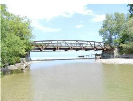
The bottom chords are completely severed at the west end while at the east they are almost completely severed. The top chords are buckled.
