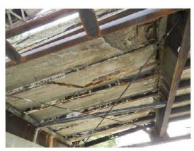
The northeast bearing seat has failed and the northeast wing wall should be partially removed as well.
