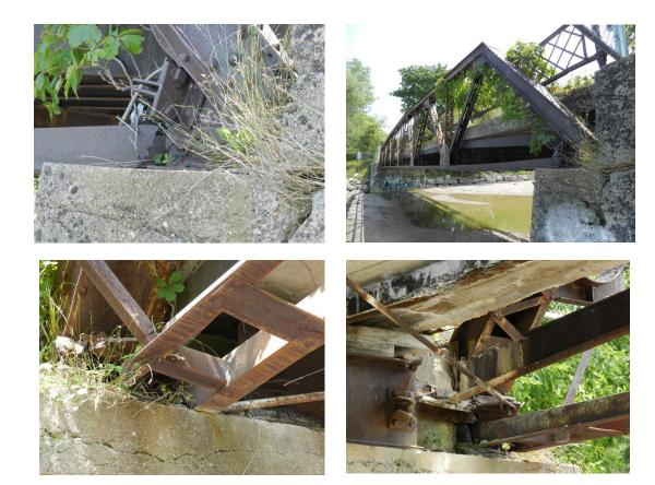
Stringers at the east end are in very poor condition as is the concrete deck which poses at the very least an overhead falling debris hazard.
